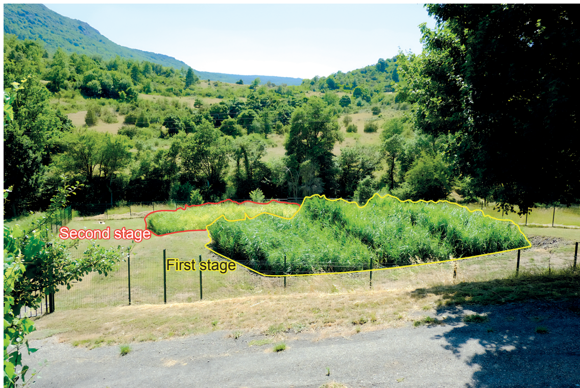
Figure 2(h): Reed bed sewage system on a tributary of the Agly river at Cubières-sur-Cinoble
